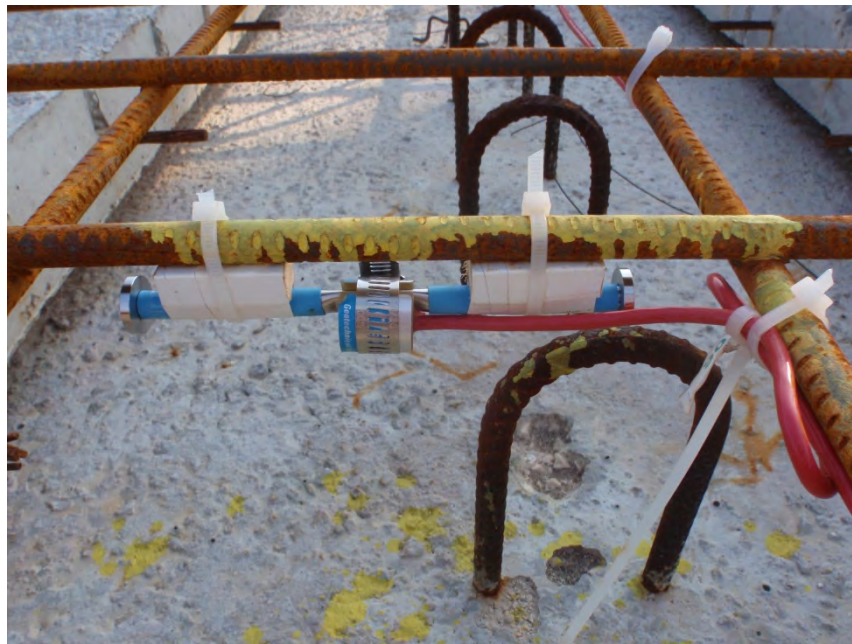
Figure 3-72: Typical field installation of VWG, Lampasas River Bridge
