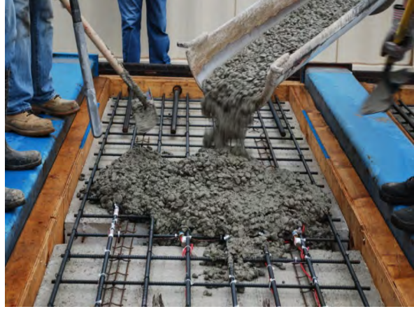
(b) Place concrete
