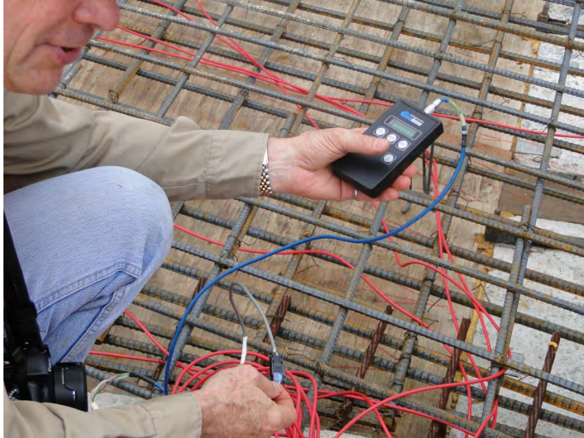
Figure 3-74: Checking gage before threading wire through the holes in bedding strip, Lampasas River Bridge
