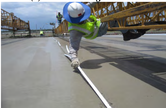
(e) Inserting crack former
