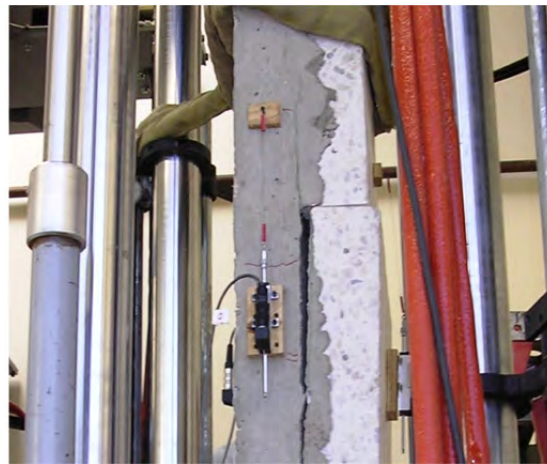
Figure 2-13: Delamination during DTT (Foster 2010)
