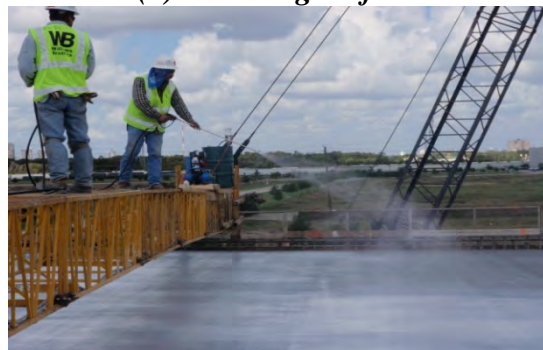
(f) Spraying curing compound on deck surface
