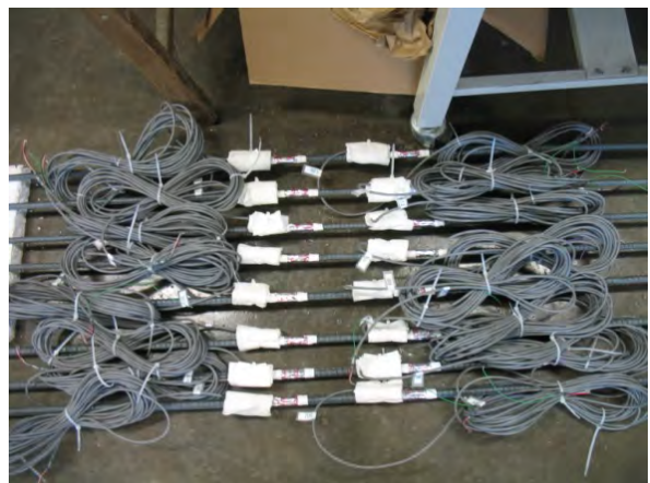
(f) Completed installation
