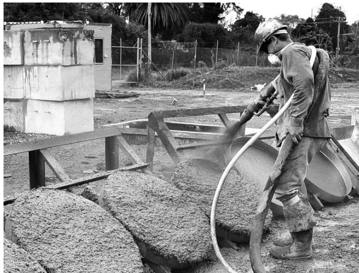
Figure E-12: Manual spraying of shotcrete panels (ASTM C1550 2010)
