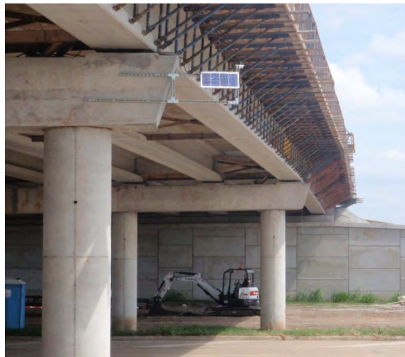
Figure 3-20: Mounting solar panel beside bent cap, Wharton-Weems Overpass
