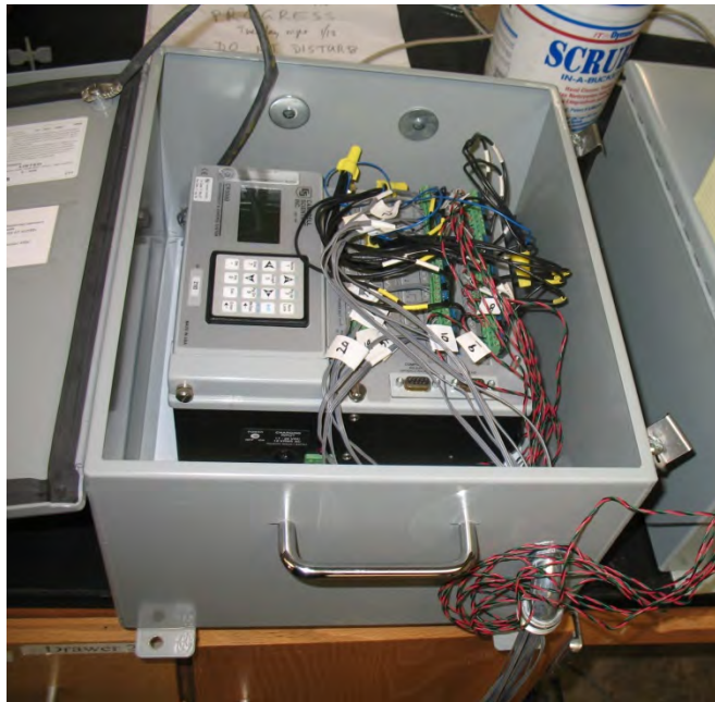
Figure 6-7: Steel box for data logger
