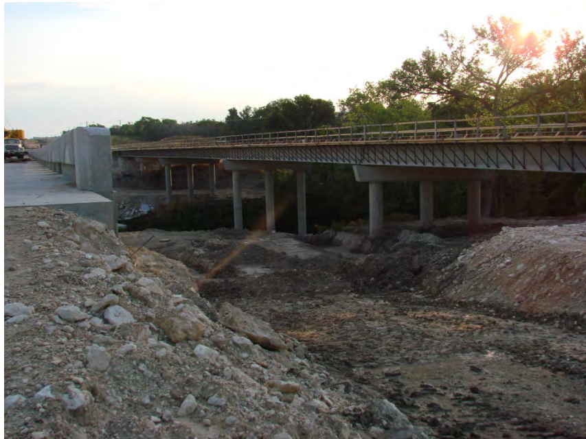
Figure 3-71: Side view of Lampasas River Bridge from south end
