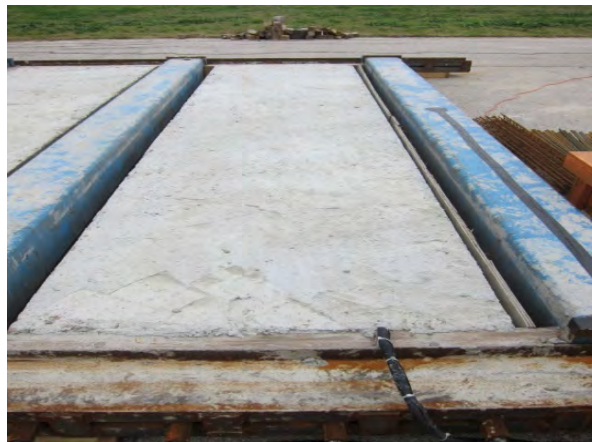
(f) Strip wooden form on one side
