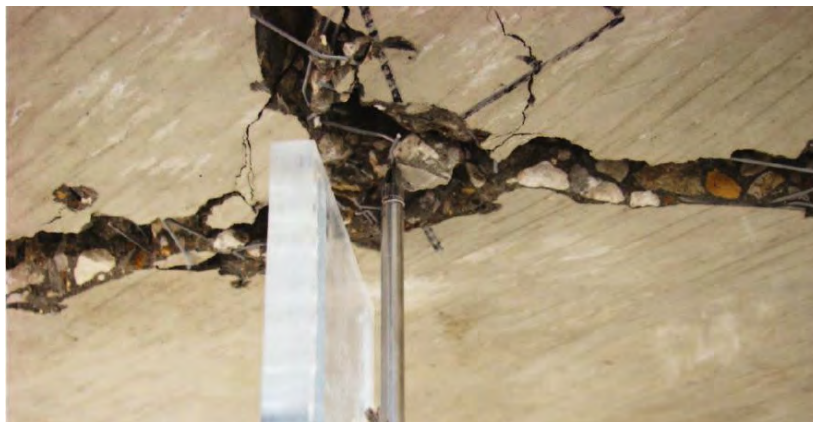
Figure E-15: View of underside of ASTM C1550 test specimen showing crack width vs. LVDT probe width at location of LVDT (S.-H. Chao 2011)
