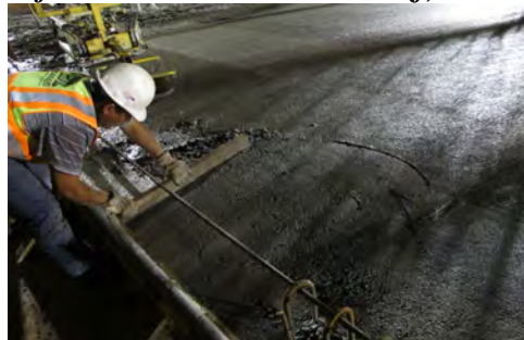
(g) Hand screeding of portion of deck
