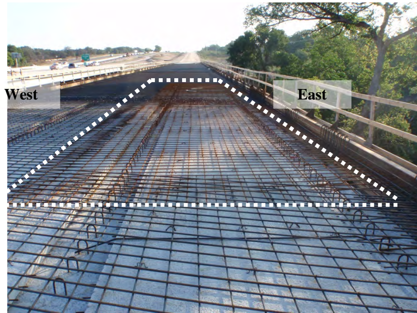
Figure 3-65: Test area for reduced welded-wire reinforcement, Lampasas River Bridge
