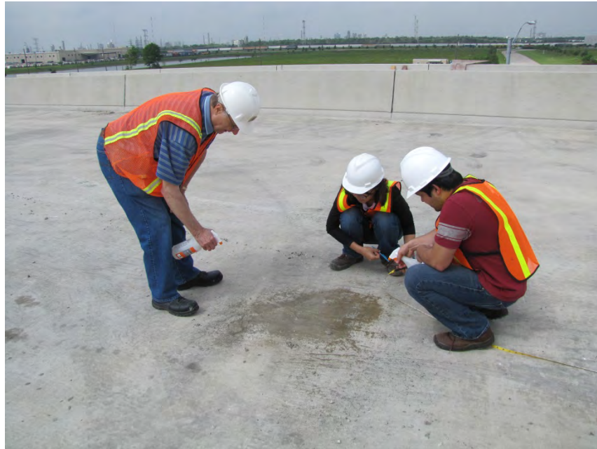
Figure 3-22: Spraying water on bridge deck for cracking inspection, Wharton-Weems Overpass
