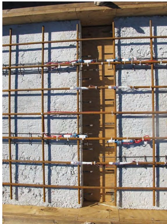
Figure 4-17: Complete gage installation for one bay of restrained-shrinkage test
