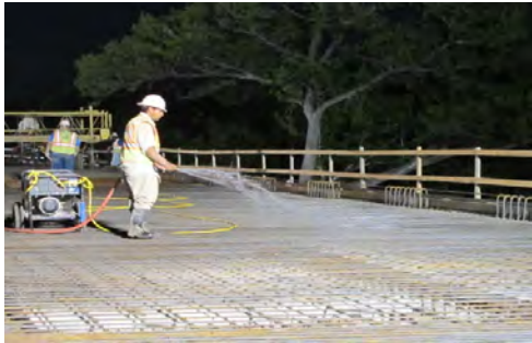
(a) Spraying water on panels
