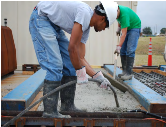
(c) Consolidate with hand-held vibrator
