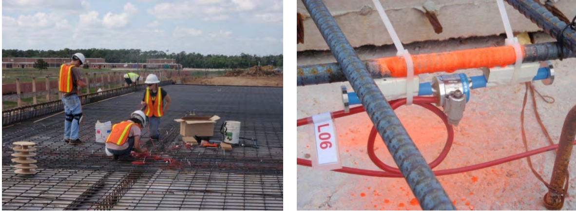
Figure 3-17: Gage instrumentation, Wharton-Weems Overpass
