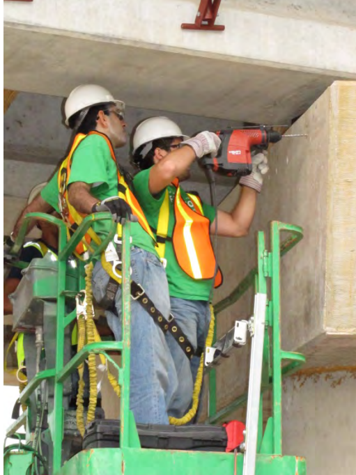
Figure 3-81: Drilling holes on the side face of the bent caps for anchor bolts, Lampasas River Bridge
