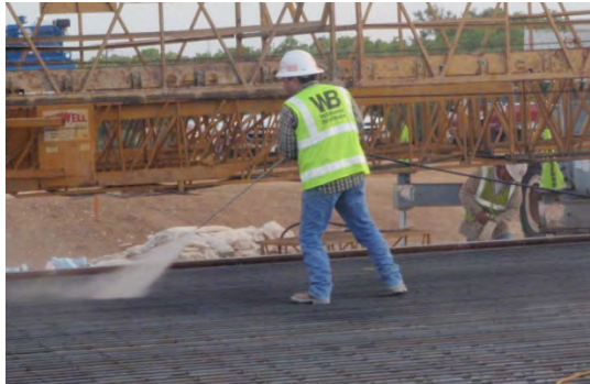
(a) Spraying water on panels
