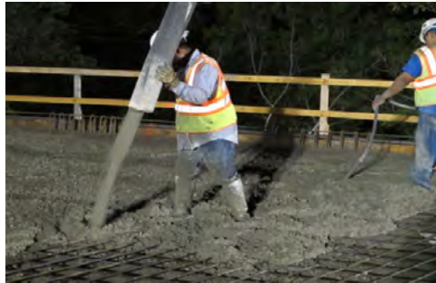
(b) Placing concrete
