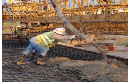
(b) Placing concrete
