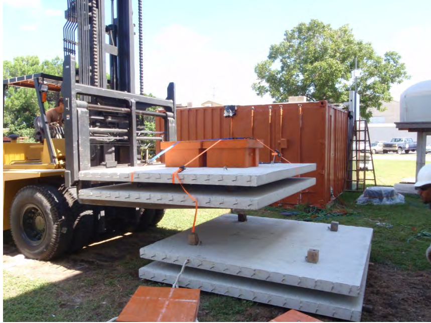
Figure 6-4: Stacking panels at Ferguson Laboratory (Azimov 2012)
