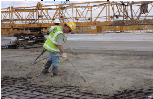
(c) Consolidating concrete
