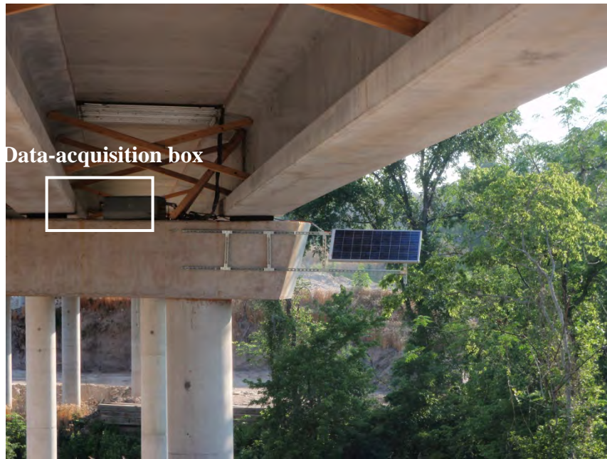
Figure 3-77: Data-acquisition box between Spans 1 and 2, Lampasas River Bridge
