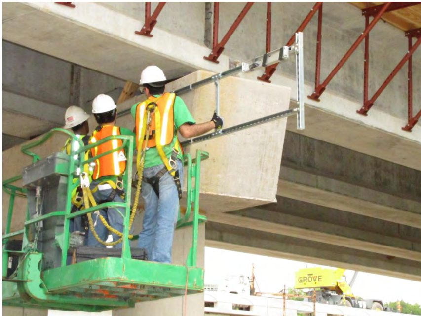
Figure 3-82: Mounting bracket for solar panel, Lampasas River Bridge
