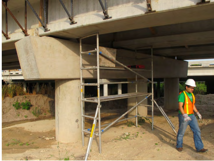
Figure 3-79: Scaffolding for accessing bent cap between Spans 4 and 5, Lampasas River Bridge
