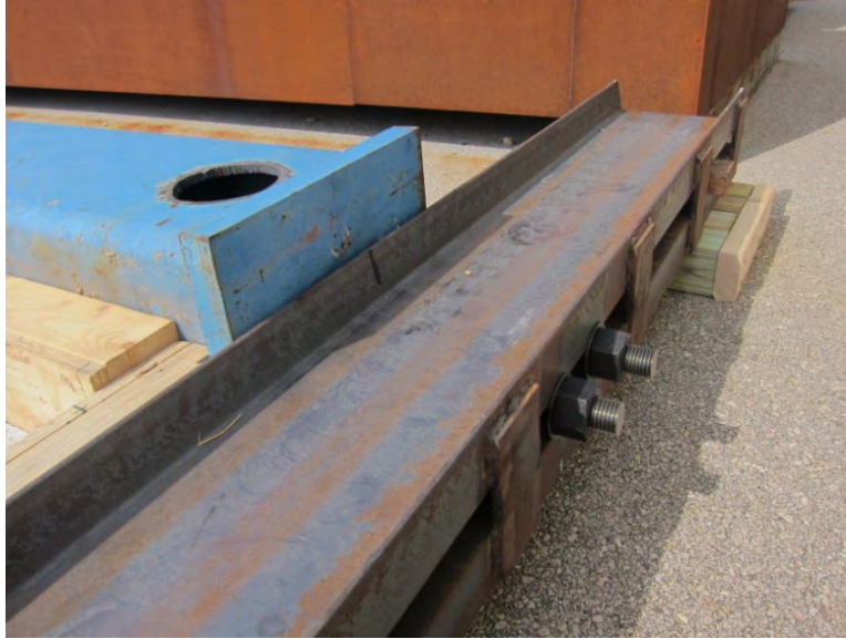
Figure 4-6: Attaching steel tube to back-to-back channels
