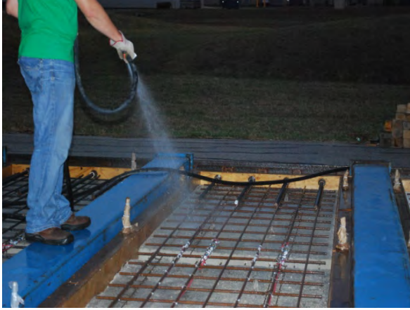
(a) Spray water on panels
