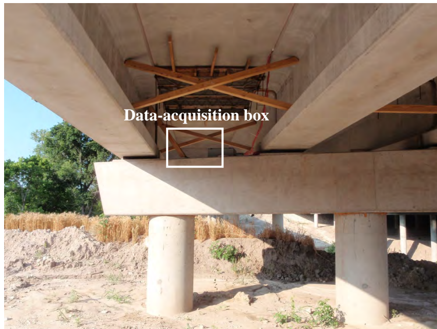
Figure 3-78: Data-acquisition box between Spans 4 and 5, Lampasas River Bridge
