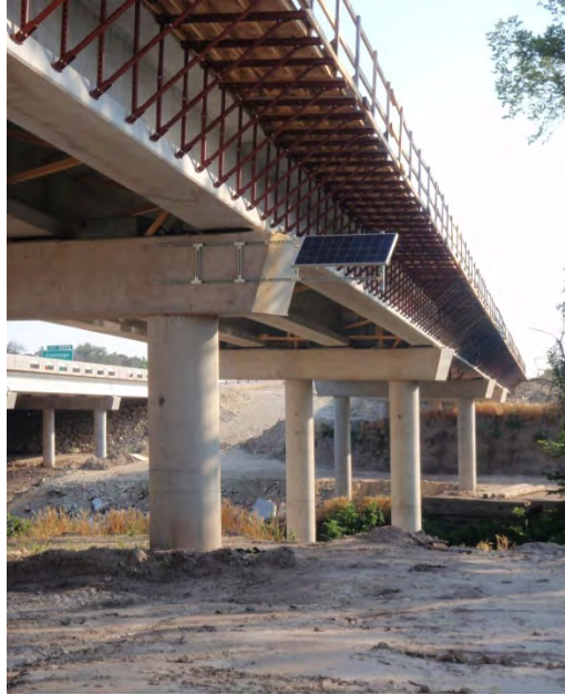
Figure 3-83: Solar panel mounted on side face of bent between Span 1 and 2, Lampasas River Bridge
