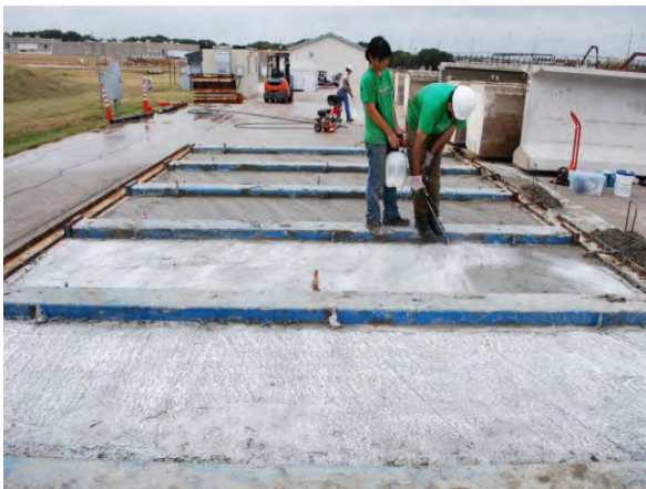
(e) Spray curing compound
