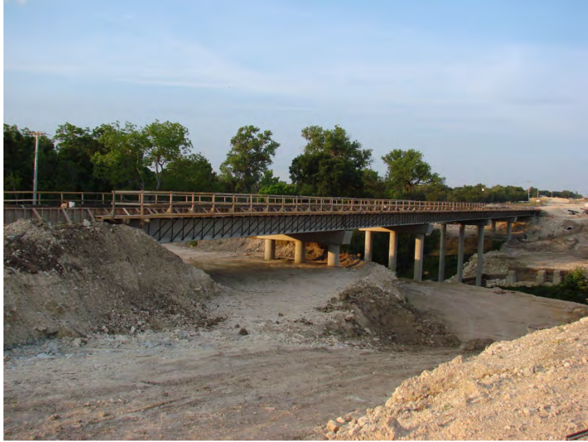
Figure 3-70: Side view of Lampasas River Bridge from north end
