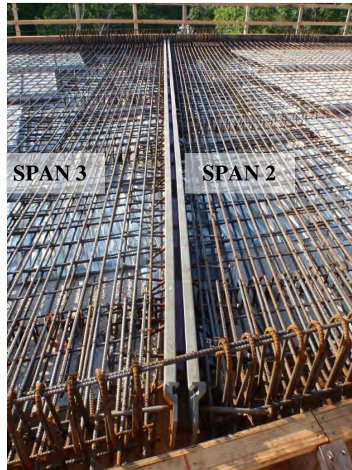
Figure 3-69: Armor joint between Spans 2 and 3, Lampasas River Bridge
