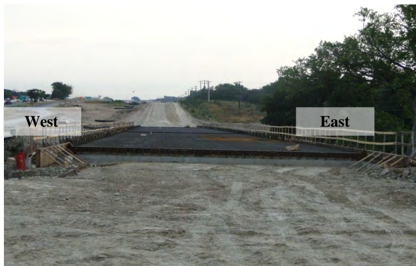
Figure 3-62: View of top-mat reinforcement from south end, Lampasas River Bridge
