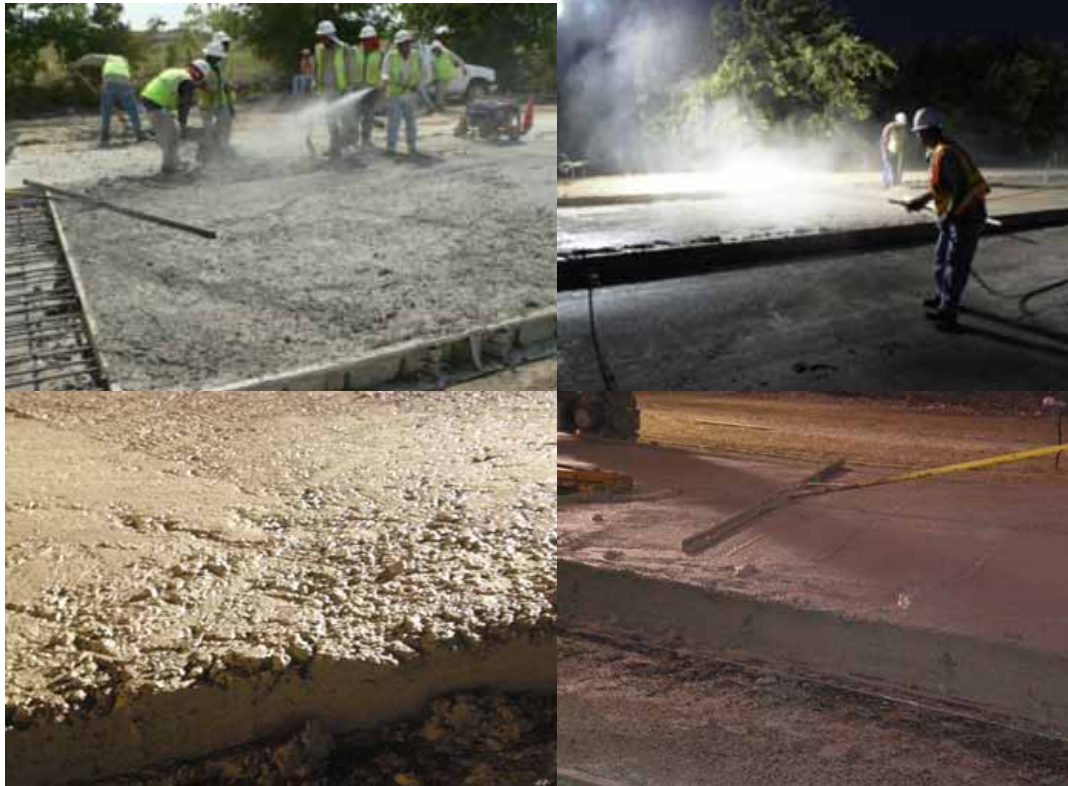
Figure 9.7: Finishability Problems Encountered with 100% MFA Sections [McLeroy, 2008]
