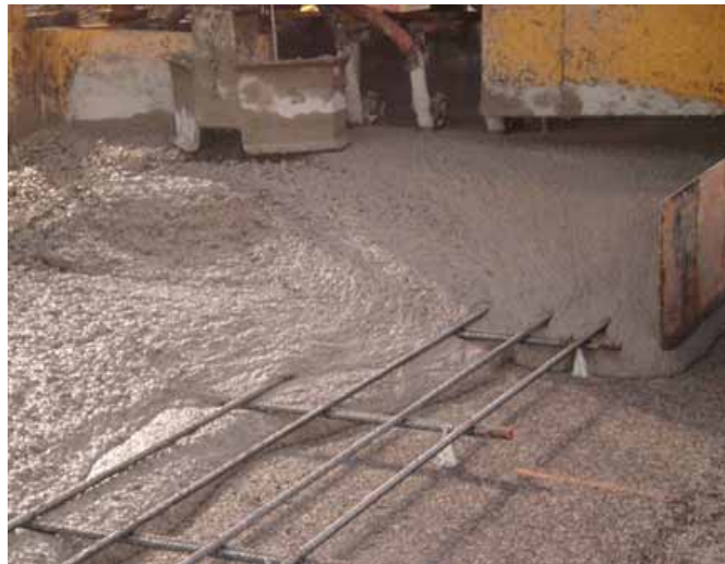
Figure 9.6: Concrete with a Slump Exceeding the Requirements [McLeroy, 2008]
