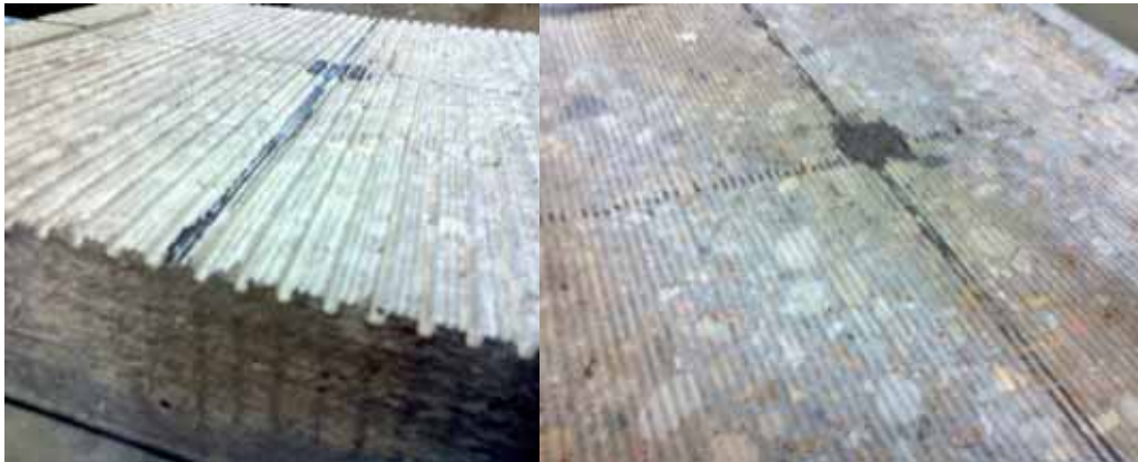
Figure 12.1: Diamond Ground Concrete Slabs
