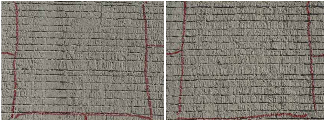
Figure 9.13: Section 4 Wheel Path (left) vs. Between Wheel Path (right)
