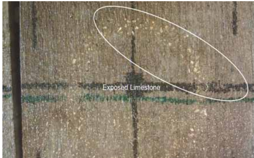
Figure 11.11: Concrete Slab with Exposed Limestone Coarse Aggregate
