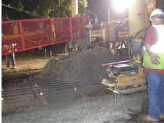
Figure 9.5: Low Slump Concrete - 5% Microfine Mixture [McLeroy, 2008]
